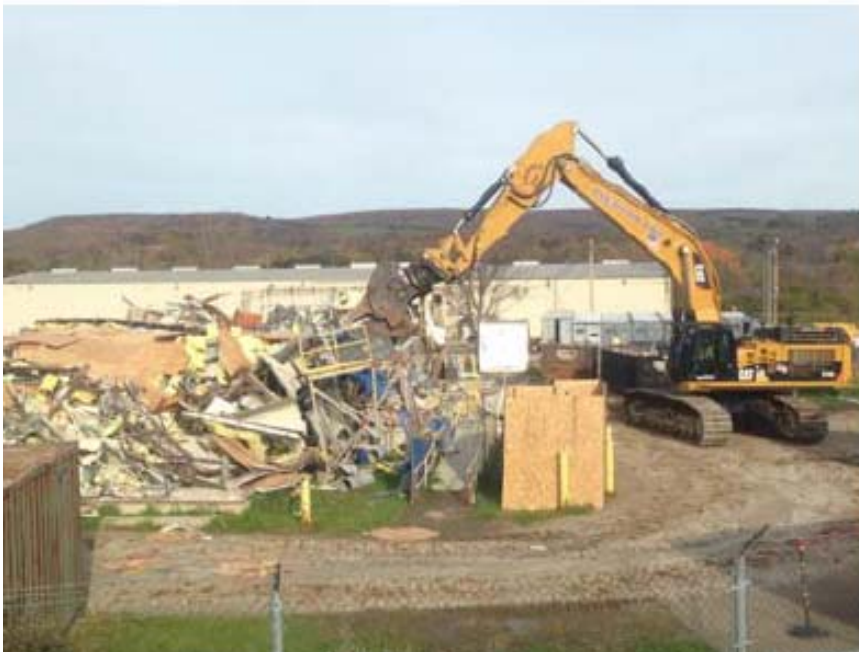
E-Lab Demolition and Waste Loadout
