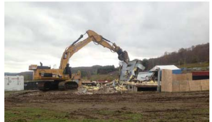
E-Lab Demolition Waste Loadout
