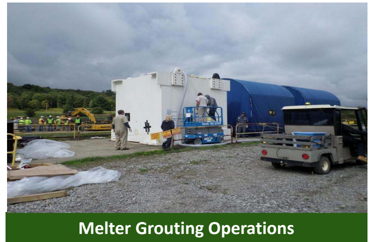
Melter Grouting Operations
